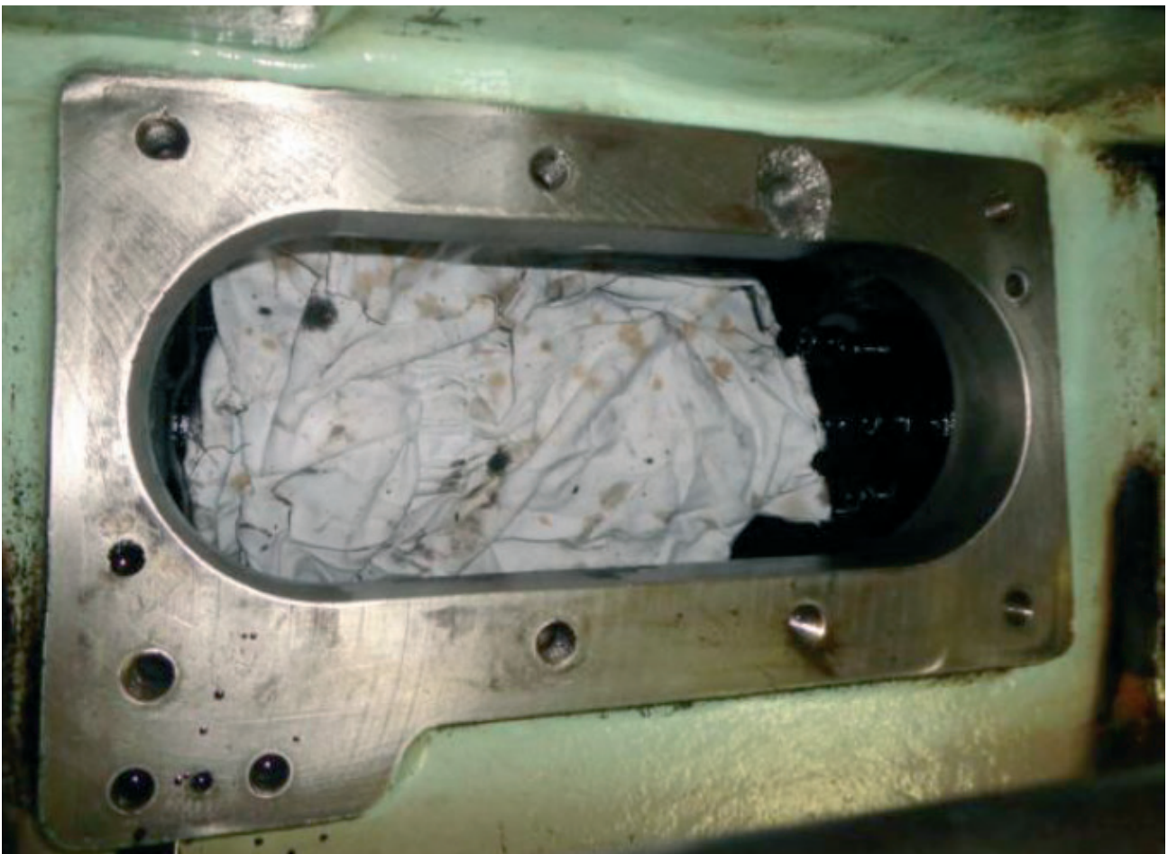
Frame surface damaged
