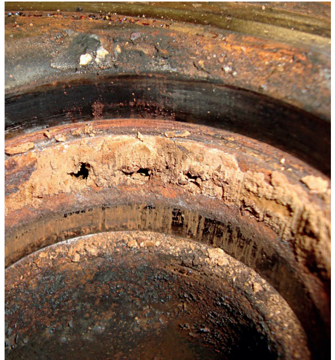
Fig. 3: Rust and limescale blocks the cooling water bores (valve seat removed from cylinder head)
