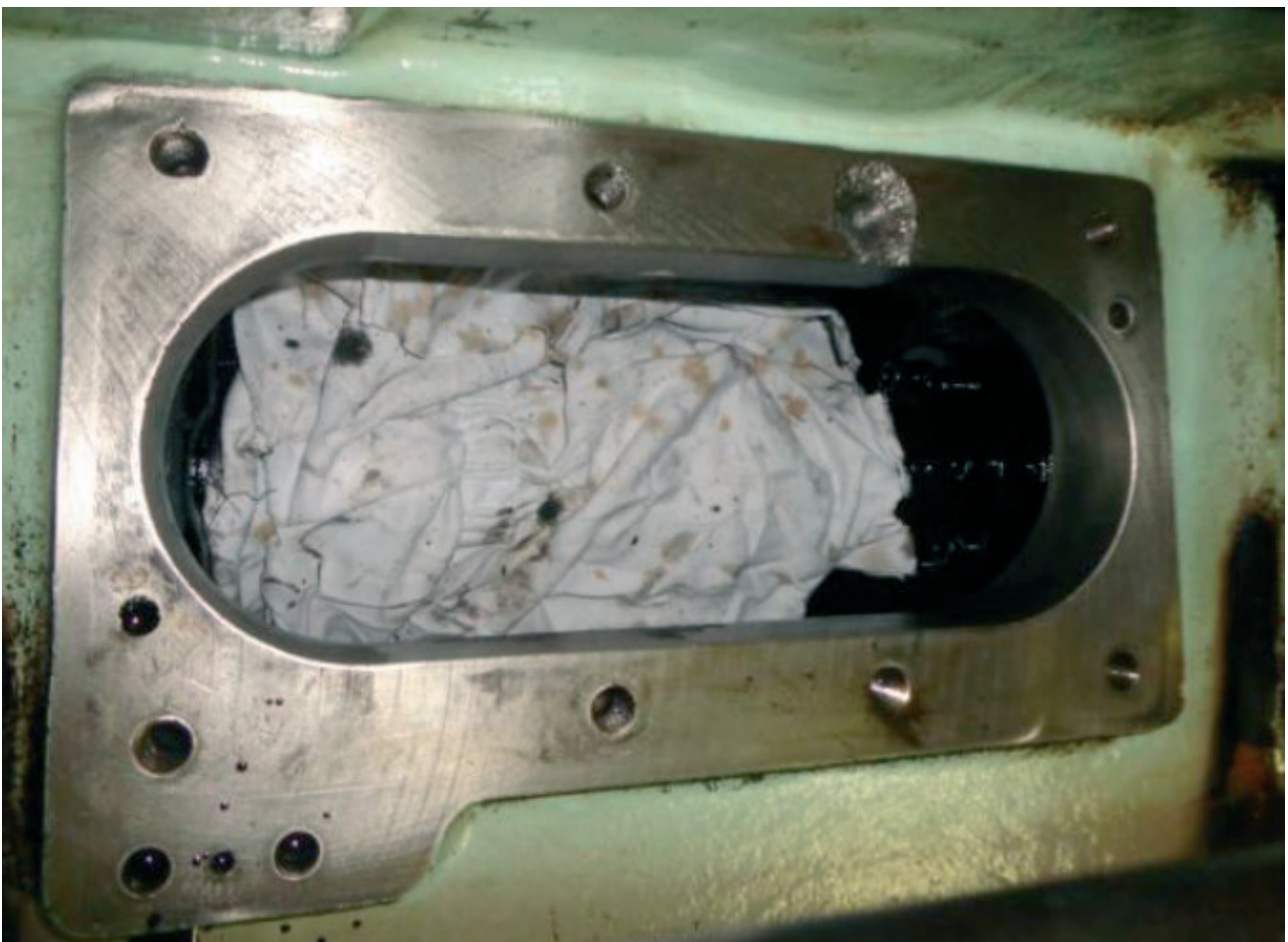
Frame surface damaged
