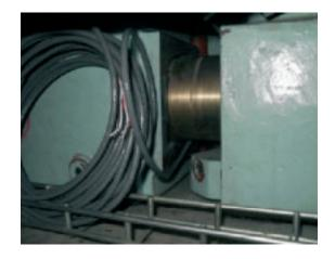
Make sure that the cable is not touching the exhaust gas pipe
