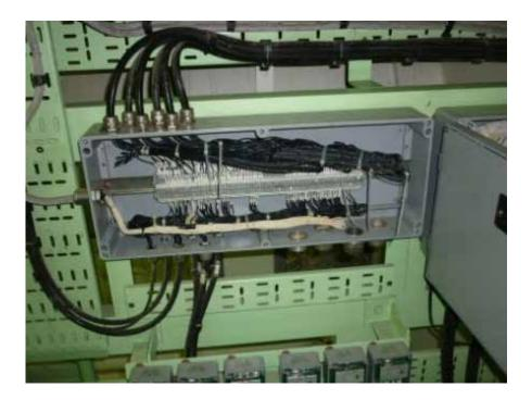
Figure 19: A junction box with a long unsupported wire bundle
