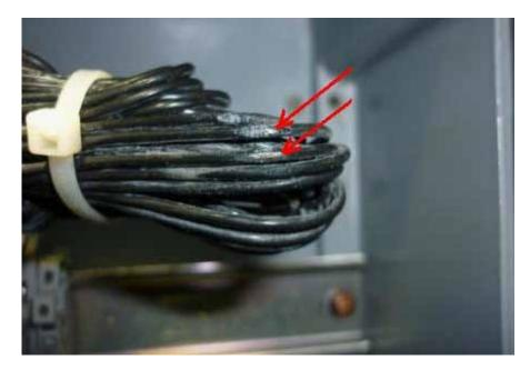
Figure 20: Red arrows indicating where the insulation was worn off.
