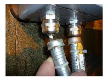
Figure 15: Cable damaged in gland to fuel plunger sensor tail junction box.
