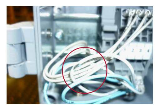
Figure 5: Examining the wires reveals that the insulation has been worn off (red circle); causing electrical noise whenever the uninsulated piece touched the side of the junction box.
