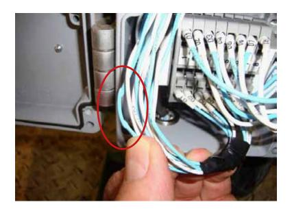
**Figure 7:** When opening the lid it can be seen that one of the wires had been pinched when the junction box was last closed (red circle); causing penetration of the insulation.
