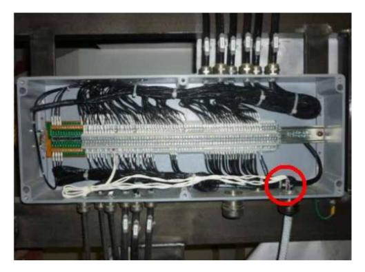
Figure 21: Junction box with a lot of unsupported wire bundles. The red circle indicates where chafing was most severe.
