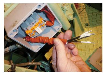
12. Fit the silicone flex tube onto the wires (max. 5 wires inside one silicone flex tube).
