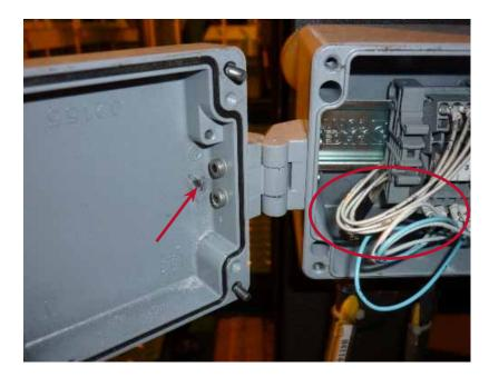
**Figure 4:** Upon opening the junction box it is apparent that the unsupported wires (red oval) have been chafing against the lid, causing a clear mark (read arrow).
