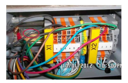
Figure 23: Unsupported wires. Leading to chafing and loss of insulation (red circle).
