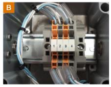
A: Chafed wires in MTBFPB: Correctly installed wires in MTBEV
