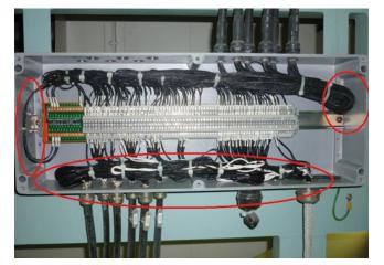
Wiring in contact with TB-LOP interior
