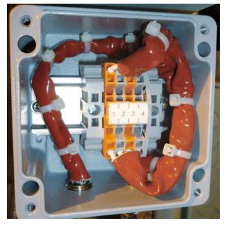
MTBEV installed with the "silicone kit"
