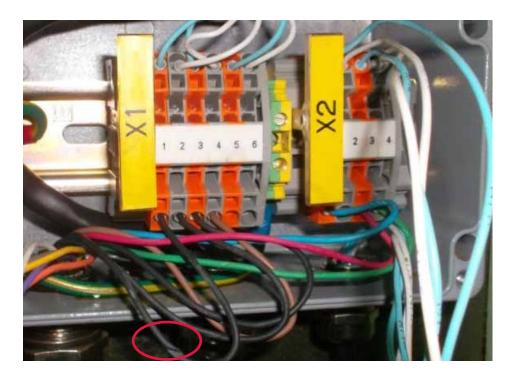
Figure 24: Unsupported wires. Leading to cables being pinched when the junction box is closed (red circle).
