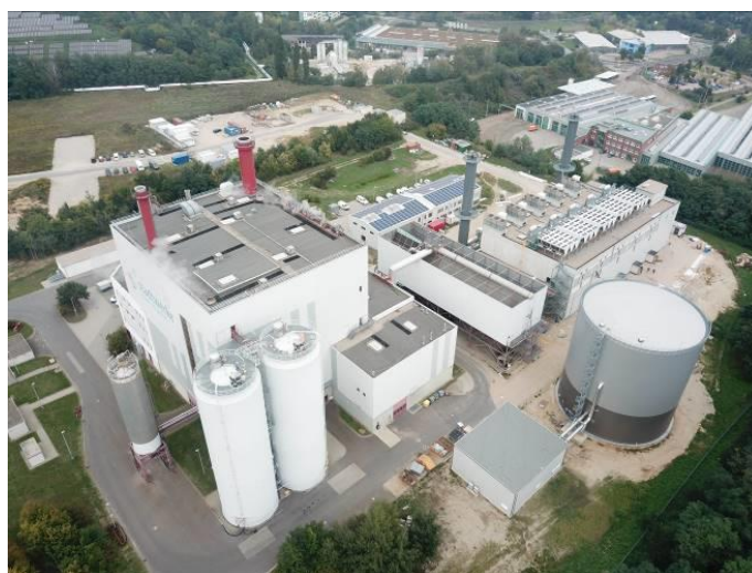
MAN Energy Solutions has commissioned the new, municipal CHP gas power-plant in Frankfurt (Oder) ©Stadtwerke Frankfurt (Oder)
