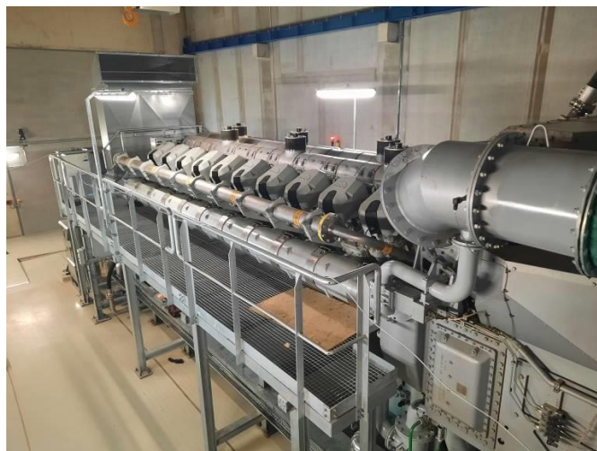
The CHP plant is powered by 5 × MAN 20V35/44G gas engines.
