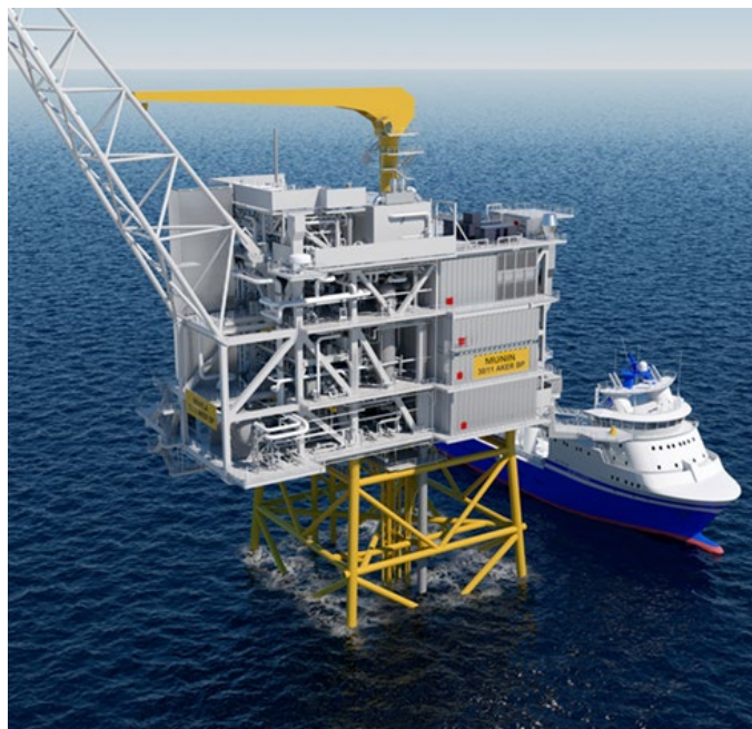
The Munin gas production platform will be remotely operated from onshore (picture ©Aibel)
