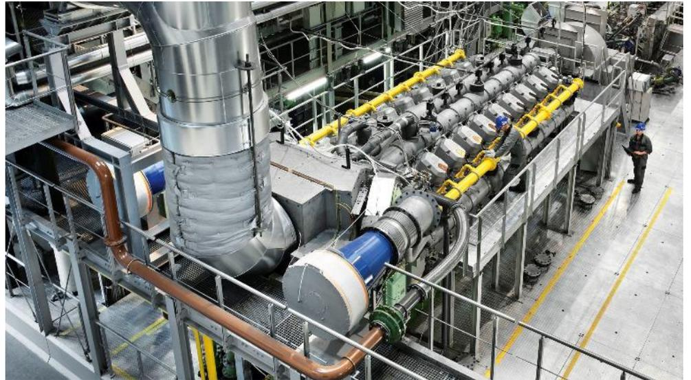
*Gas-powered, four-stroke engines from MAN Energy Solutions are operable in stationary mode with a hydrogen content of up to 25% by volume in a gas-fuel mix.*
