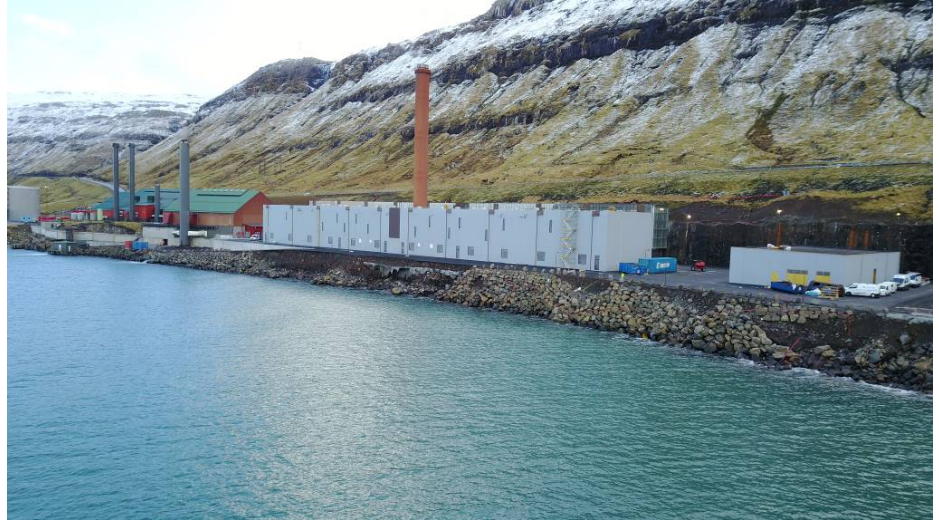
MAN Energy Solutions has completed the expansion of the 'Sund' power plant near Tórshavn, the Faroese capital.
