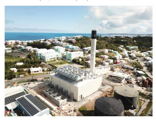
Four MAN 14V51/60DF engines extend the power plant complex in Pembroke, Bermuda, adding another 56 MW to the island's grid
