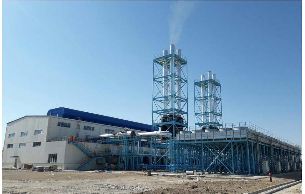
*Six MAN 18V32/40 engines form the backbone of a power plant that will generate around 54 MW of electrical energy for a new cement plant in Samawa, Iraq.*
