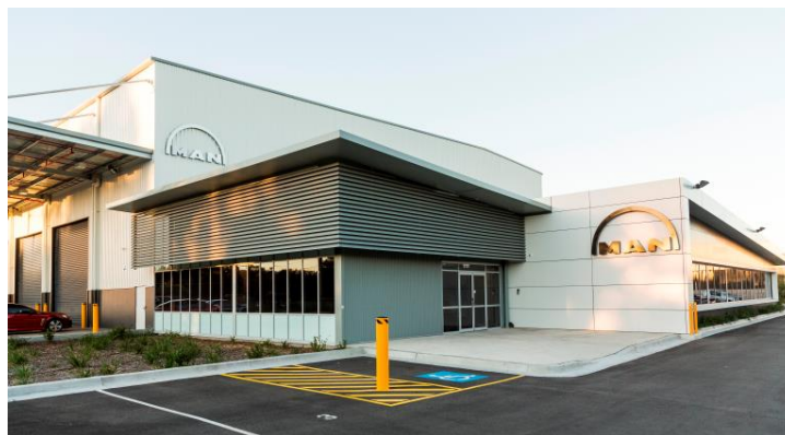
MAN Energy Solutions' new building in Sydney, Australia
