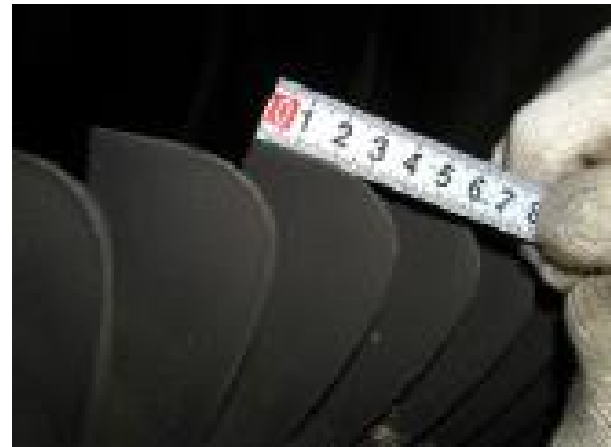
Worn turbine blade tips
