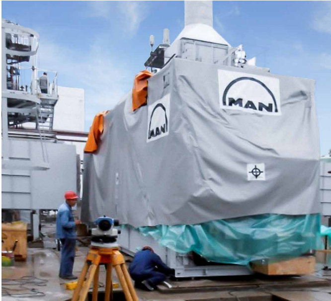
Picture 2: Installation of the gas turbine packages on site in Shanghai
