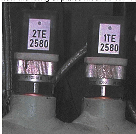
Fig. 18: Sensors with glued on aluminium plate
